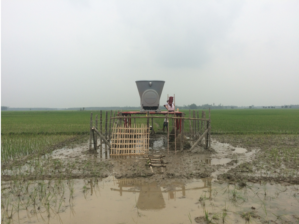
Looking in from North
